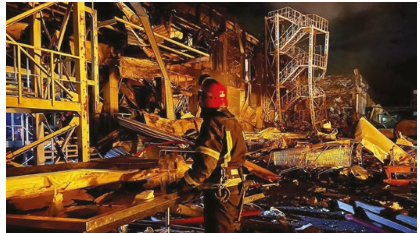
Rescuers working at the site of a missile strike in the southern Ukrainian city of Odesa in May, 2022. The State Emergency Service of Ukraine said that a shopping centre and three warehouses were hit by shelling. See p52 for the CRJ's feature on Ukraine State Emergency Service of Ukraine | Shutterstock
